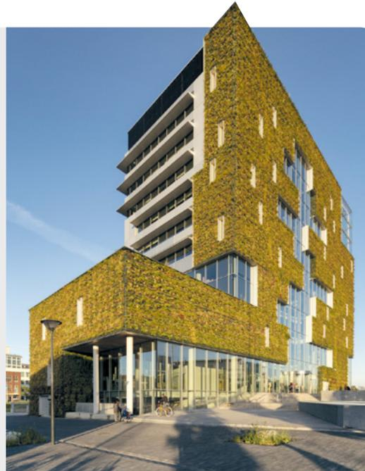
dismantled. There are several cycles in the building. The south façade is constructed using aluminium and is fully reusable without losing any of its value. The biological north façade consists largely of plants and greenery.
